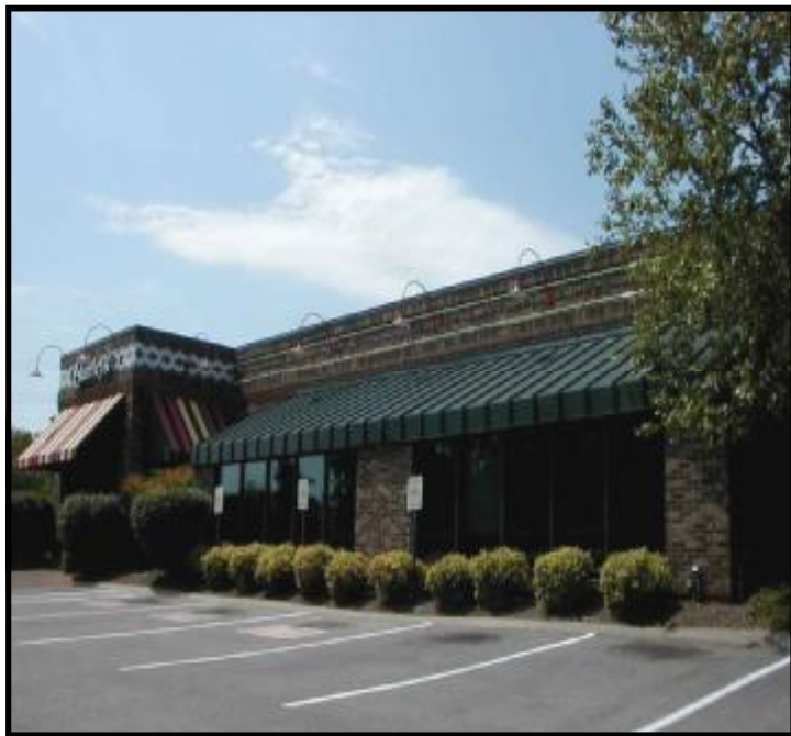
South Side of Property
